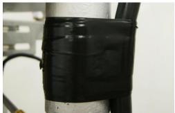
4. Ensure there is at least a 4 to 5 foot (1.5 meters) separation between taping sections per NEC.
