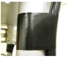
2. Wrap three full turns of one-inch Scotchrap Filament #890 tape, or the equivalent, over the Scotchrap #50 tape.
