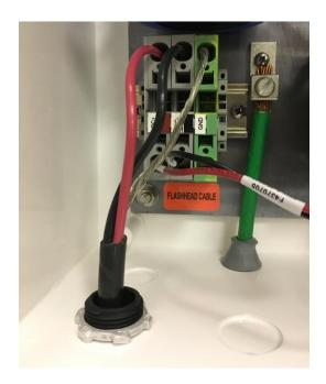
Figure 2-5 – SC 370 Flashhead Cable Connection **Securing the Cable: 2-3-4 Tape Method** Flash Technology provides the material for securing the flashhead cable to a skeletal structure with the following technique.
