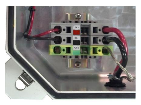
Figure 2-8 – Flashhead Cable Terminal Block
