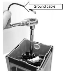
5. Using a ½ in. hex socket, remove the battery retention bolt holding down the ground cable. Remove the ground cable and recycle. Reinstall the battery retention bolt and hardware; tighten to 200 in. lbs.
