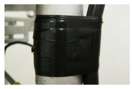
**4.** Ensure there is at least a 4 to 5 foot (1.5 meters) separation between taping sections per NEC.
