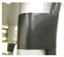
2. Wrap three full turns of one-inch Scotchwrap Filament #890 tape, or the equivalent, over the Scotchwrap #50 tape.
