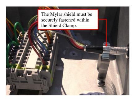
Figure 2-6 - FH Cable Shield Clamp
