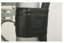
4. Perform steps 1 through 4 also directly above and below any tower leg flanges that the cable may cross. The cable should be spaced approximately 1 inch from the edge of each flange.
