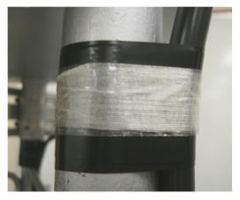
3. Wrap four full turns of two-inch Scotchwrap #50 tape, or the equivalent, over the Scotchwrap Filament #890 tape.
