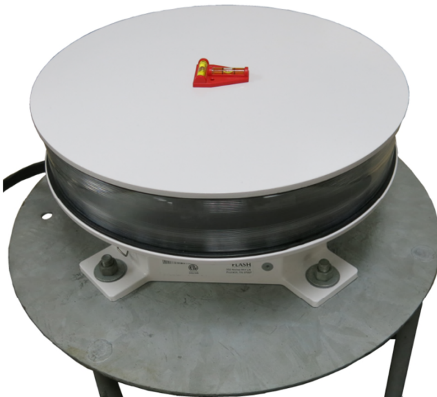
Figure 2-2 – Beacon Leveling
